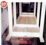
Check that the width of the two A and two B-type framed shelves will sit in their respective positions on the end frames, allowing for their relationship to the backboard rebates and the thickness of the doors
